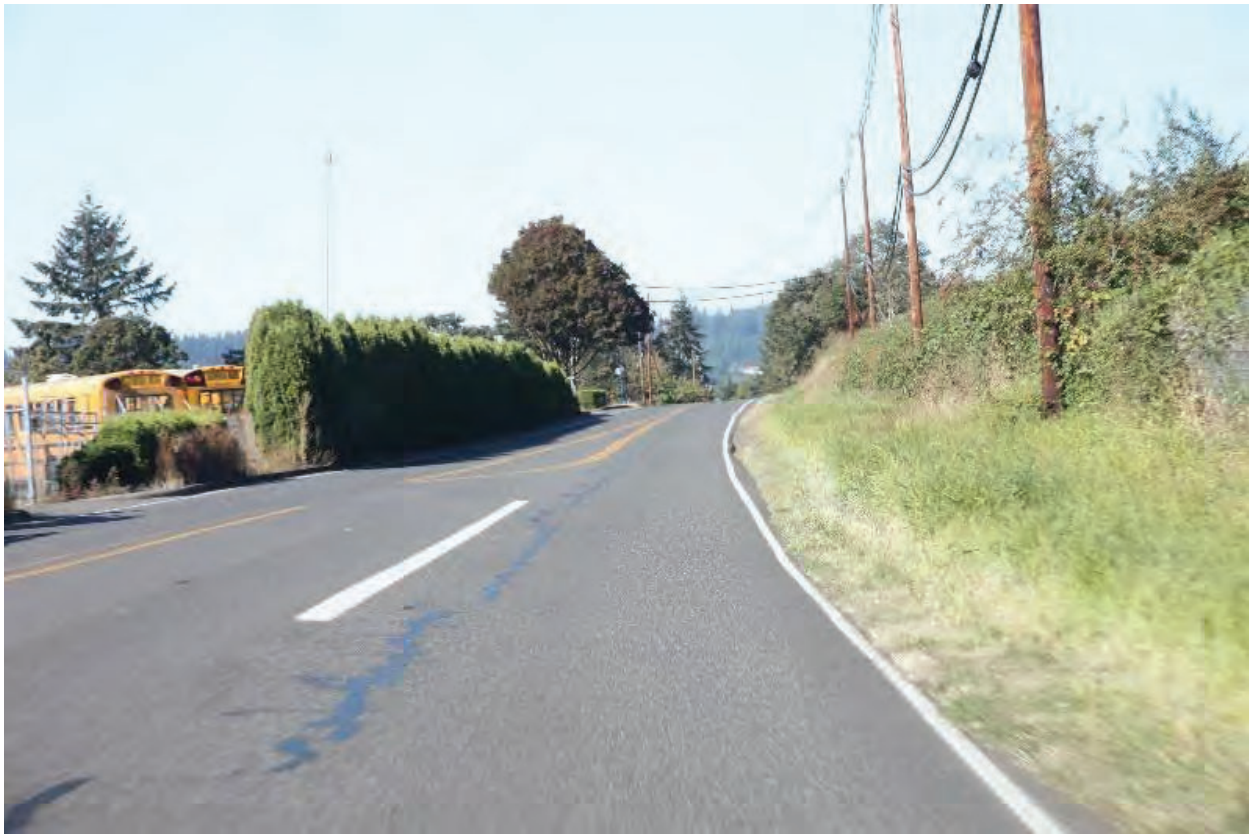
Figure 4. Existing Willamette Falls Drive Roadway Conditions
